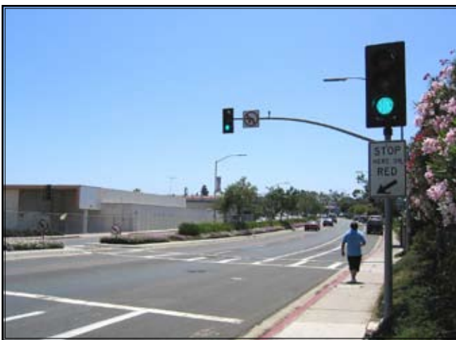
13S) This mid-block pedestrian activated crosswalk in Linda Vista includes standard traffic signals, ladder style markings, signage and a median refuge. Photo credit: Mike Singleton
