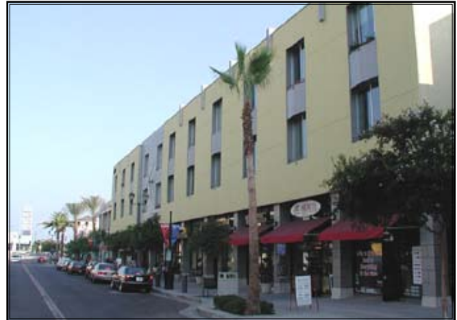
5C) The proper pedestrian environment can support a variety of retail businesses and mixed land uses while offering a pleasant urban design. Photo credit: Dan Burden
