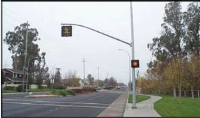
11S) This signal uses both a pedestrian crossing symbol as well as a red light when actuated. Photo credit: Michael Ronkin
