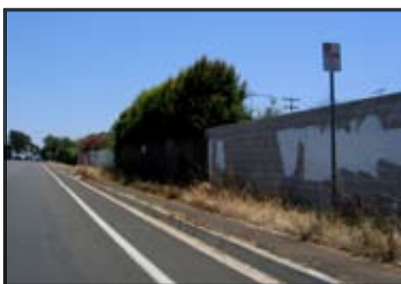
Maintenance should also include graffiti removal and vegetation control (which will limit cracking as well, especially in asphalt).
