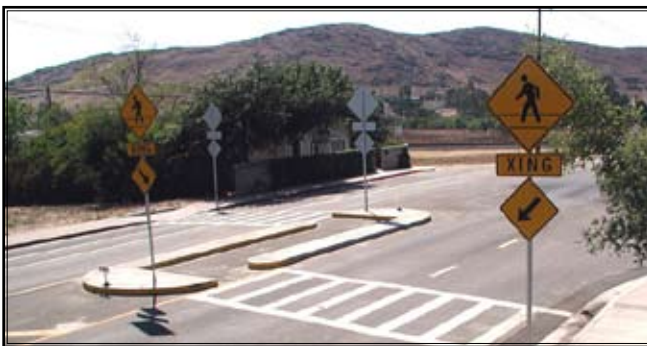
1S) Median refuges are essential where mid-block crossings are contemplated. They can include a straight cut-through or a staggered or coral style crossing. Photo credit: Dan Burden
