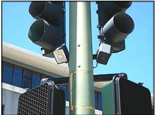
2A) Accessible and audible crossing pedestrian heads are required on most major intersections in San Diego. Audible signals do need to meet warrants. Photo credit: Dan Burden
