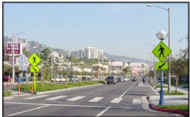
5S) Adequate lighting, pop-outs, the latest MUTCD approved signs and high visibility markings are essential for non-controlled multi-lane mid-block crossings. Note the stop bar should be located at least 30 feet from the actual crosswalk (see image on right). Photo credit: Michael Ronkin
