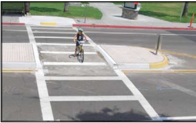
1S) A good example of a median refuge that provides access without ramps and protects a walker unable to make it across. Photo credit: Andy Hamilton
