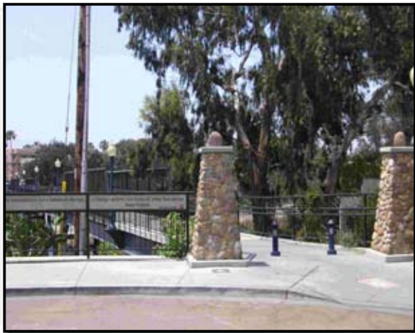
Vermont Street bridge (over Washington Street)
