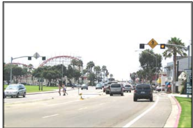
10S) A number of flashing pedestrian crossing warning signs are used in San Diego. Other solutions may be more appropriate where multi-lanes of travel on high volume streets exist. This crossing has visible signage and crosswalks along with a median refuge. Improved street lighting and advance stop bars could increase safety, but a pedestrian actuated traffic signal would provide for the safest condition. Photo credit: Mike Singleton
