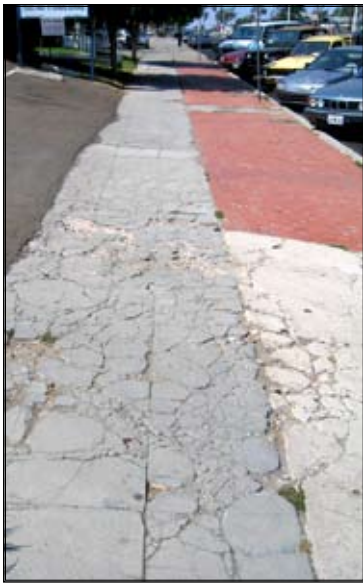
Walkways can deteriorate quickly once surface cracks have formed and water / weather changes leverages these cracks apart.
