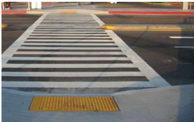
3S) Certain urban areas (that are pedestrian dominant) should utilize high visibility markings in the entire intersection. Photo credit: Michael Singleton
