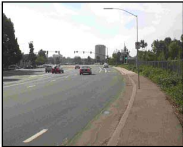
Asphalt sidewalk along curb (Genesee Avenue north of Regents Road)
