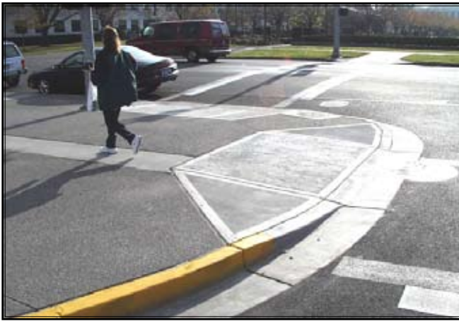
1A) Typical Two Directional Curb Ramp (note: tactile strips and truncated domes needed but not shown) Photo credit: ITE Pedestrian Bike Council
