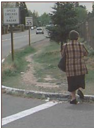
Roadway edges that were thought would never be used by pedestrians, are often used even without proper walkway facilities.
